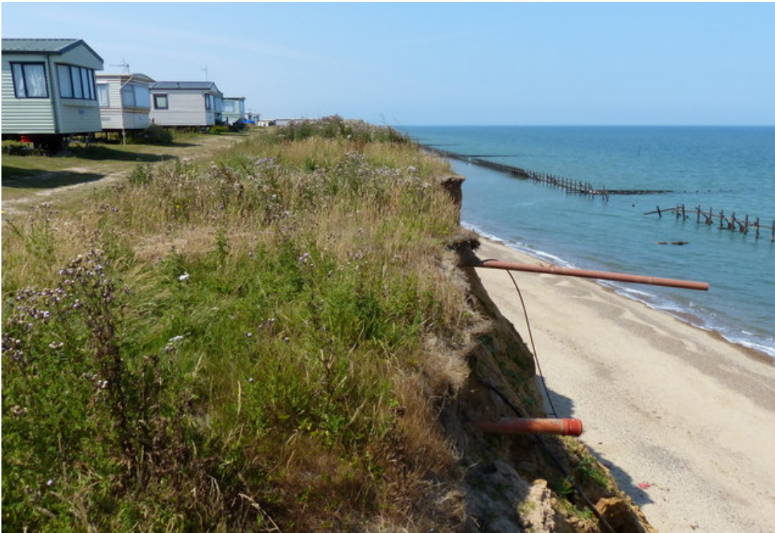
Erosion at the Happisburgh Caravan Park, ©Mat Fascione
